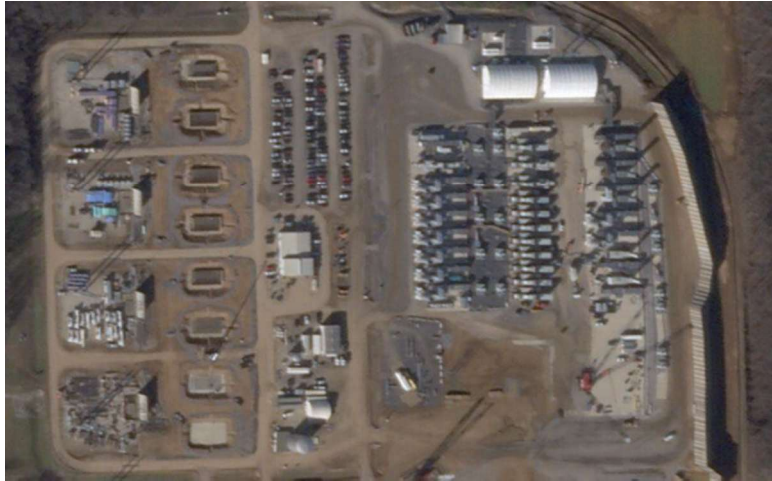
Figure 3. Close-up aerial image of xAI’s Stanton Road S. facility showing 27 turbines (Feb. 9, 2026).
