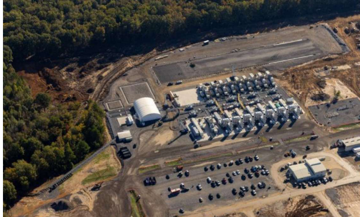
Figure 1. Aerial view of xAI's Stanton Road S. facility (Oct. 31, 2025; Steve Jones/SouthWings).
