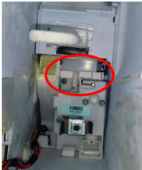
Auger Fan Blocked by Styrofoam
