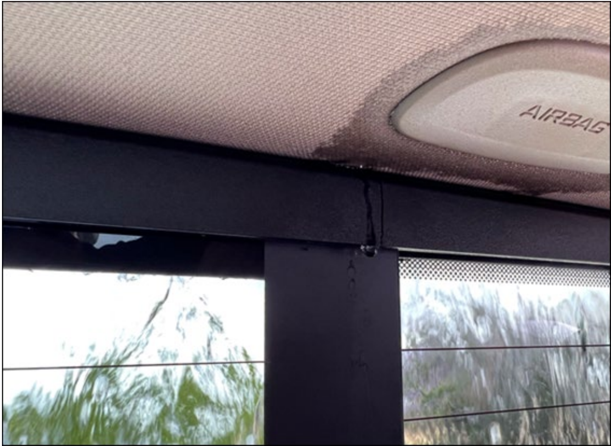
Rear facing, interior image of Plaintiff's rear cabin leaking water.
