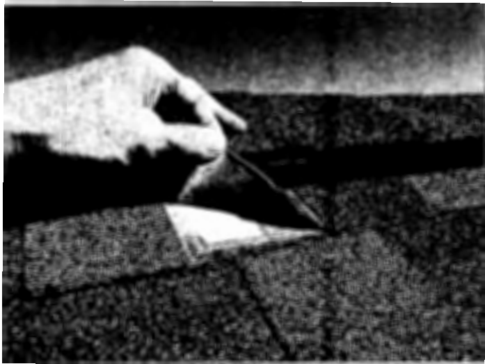
Photo 4 depicting delamination in Shingles.
