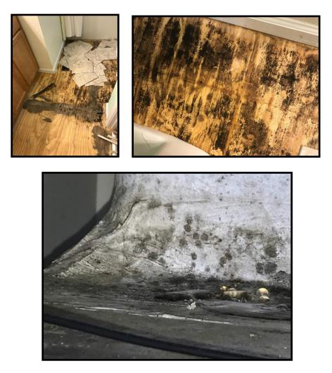
107. The window in the master bedroom became an increasing concern.<sup>86</sup> The windowsill rotted so that it could be moved and lifted, and the mold was clearly visible. When
