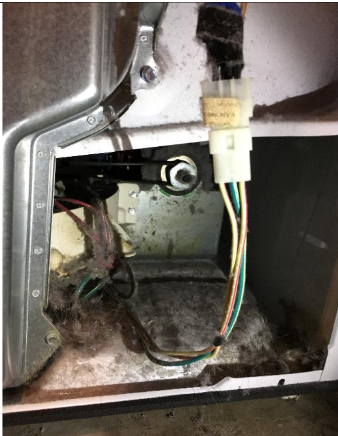
Bottom Right Side of Dryer/Disassembled After October 17, 2016 Fire
