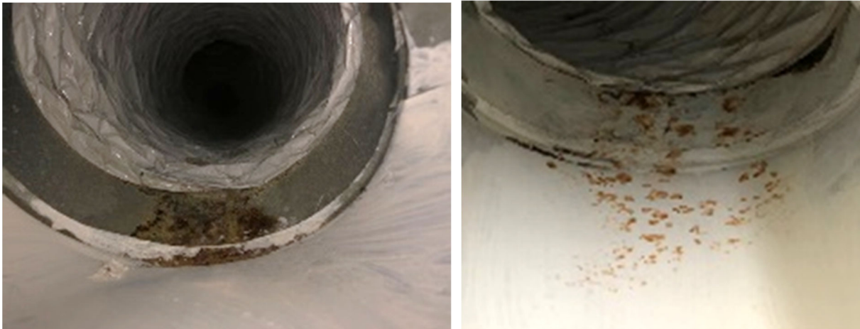
Photographs 45 and 46: Inside of Ducts
