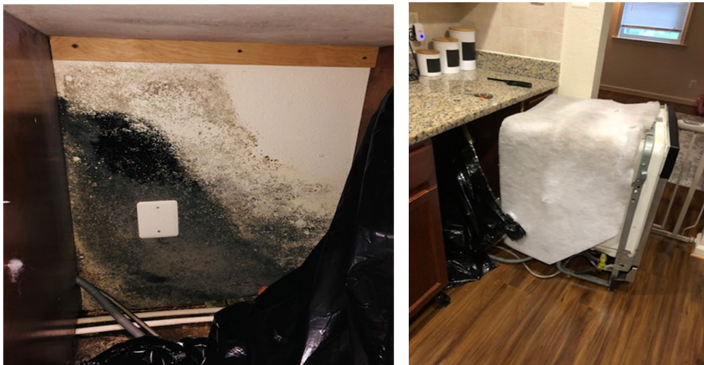
Photographs 22 and 23: Mold Behind Dishwasher
