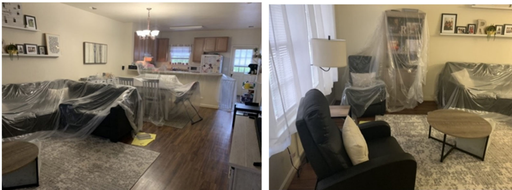
Photographs 43 and 44: Improper Containment
