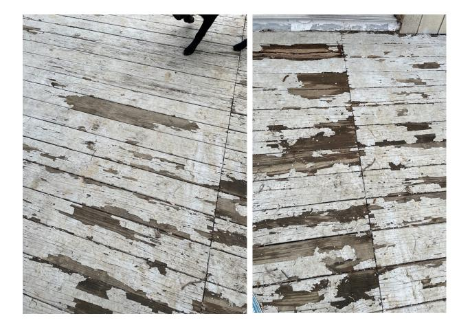
76. To date, Plaintiff's deck remains in a state of disrepair, as the Restore Products still crack, chip, strip, and otherwise fail and degrade. Plaintiff called Rust-Oleum to complain about the product failure, and Rust-Oleum failed to extend her any refund, product replacement, or
