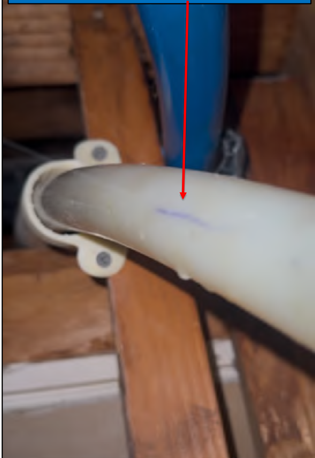
Image 7- Representative cracked and leaking Uponor PEX white pipe away from fitting
