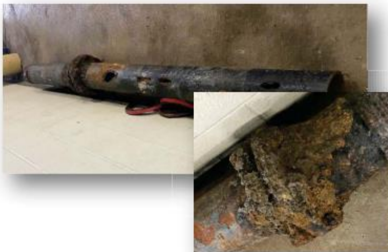
Corroded and damaged water mains
