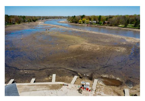
40. The Sanford Dam was next in line and also failed, resulting and expanding the flood area that reached all the way to Midland and beyond.
